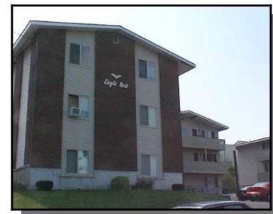
17 unit apartment building 144,150,154 Polk Street
